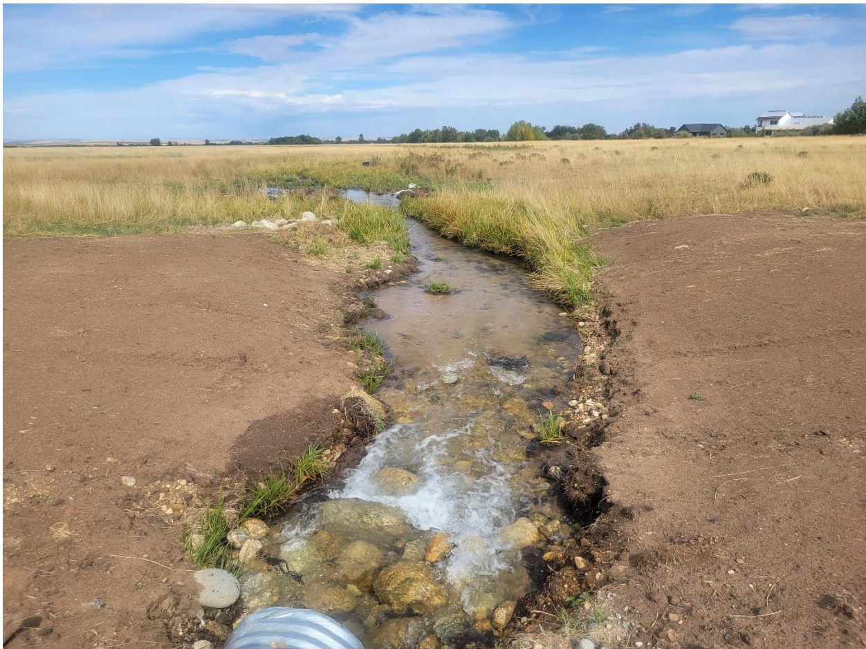
Drainage on East Side of the Subdivision
