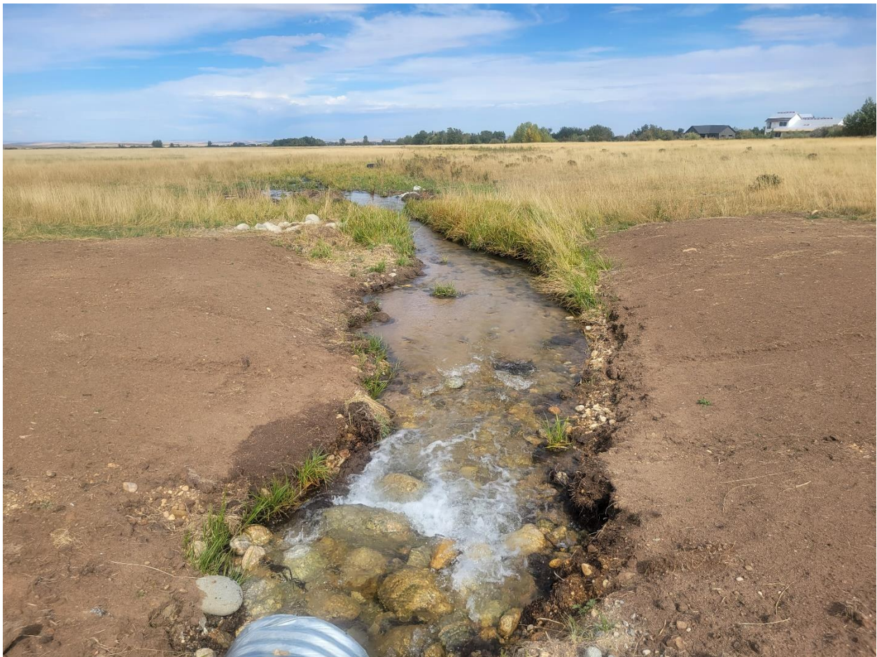
Drainage on East Side of the Subdivision
