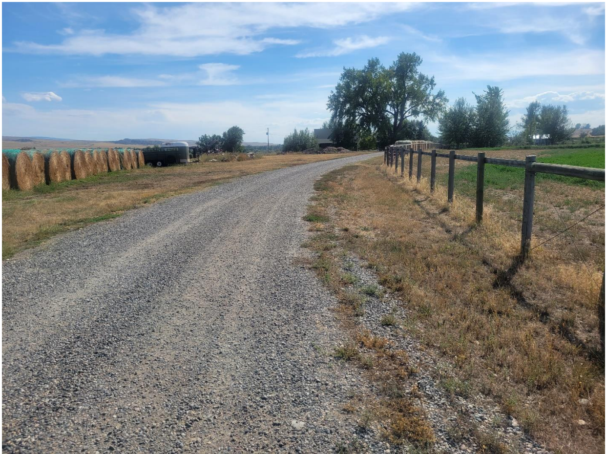
Access to Subdivision
