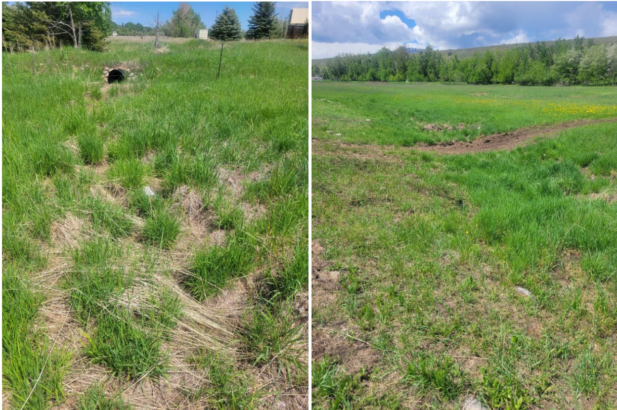
Low Areas on North Side of Subdivision
