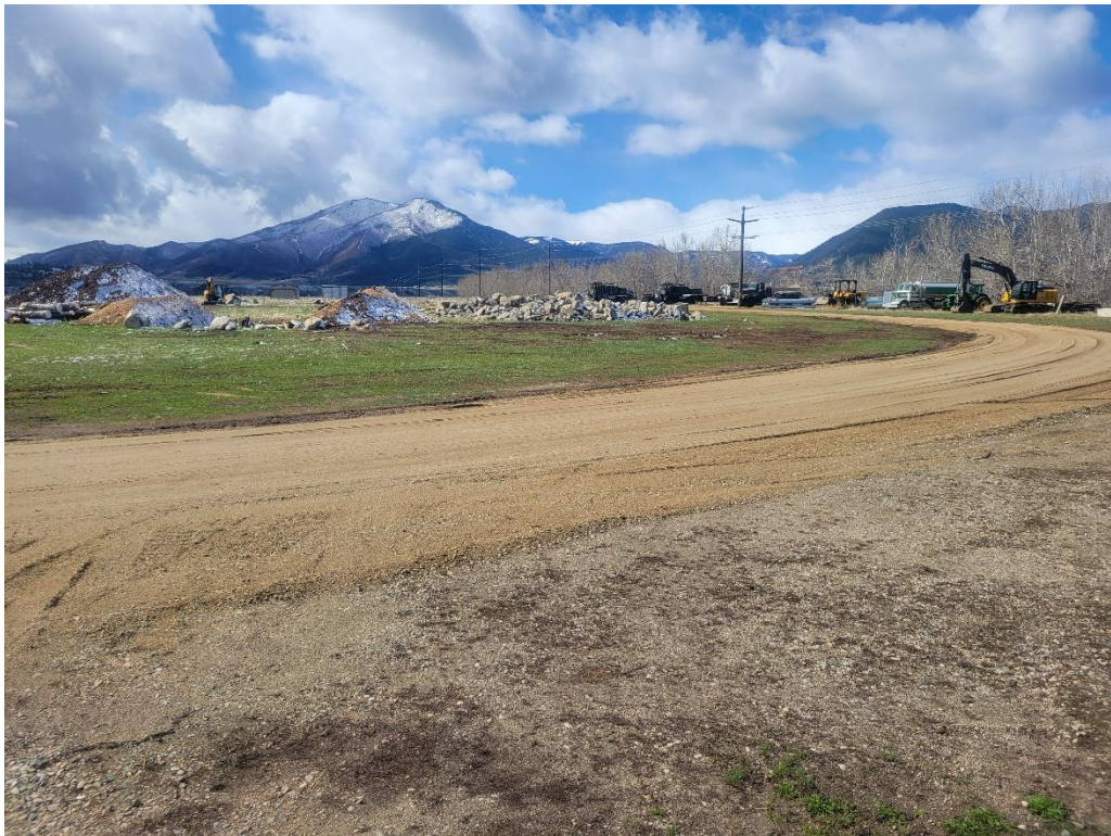
Current Equipment on Site
