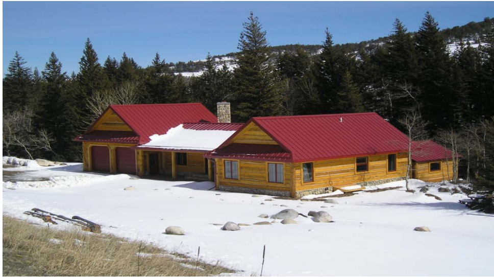
Figure 5-14. Picture of typical new construction in wildland area - log with metal roof.
