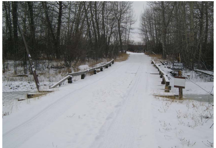
Figure 5-3. Picture of access across Rock Creek to Western Ranch Estates Subdivision
