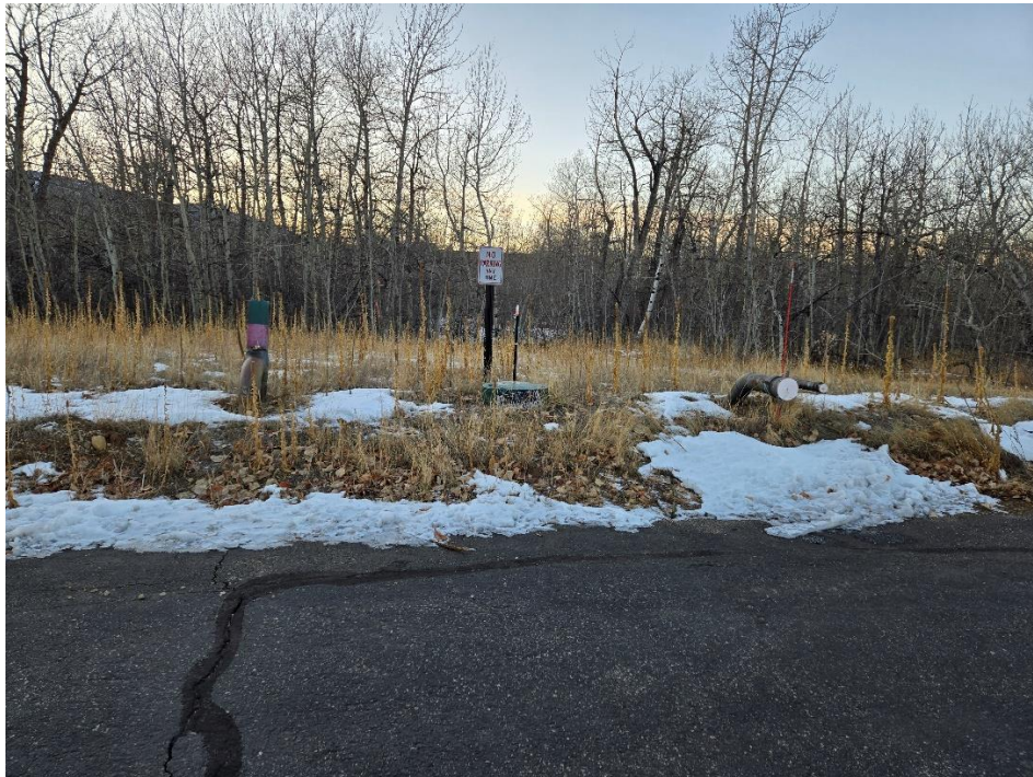
Existing Dry Hydrant
